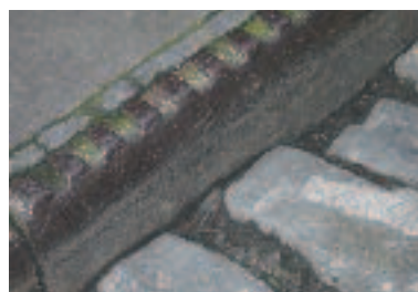
Traditional cast iron kerb
