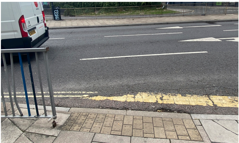
Tactiles indicate crossing where no crossing exists
