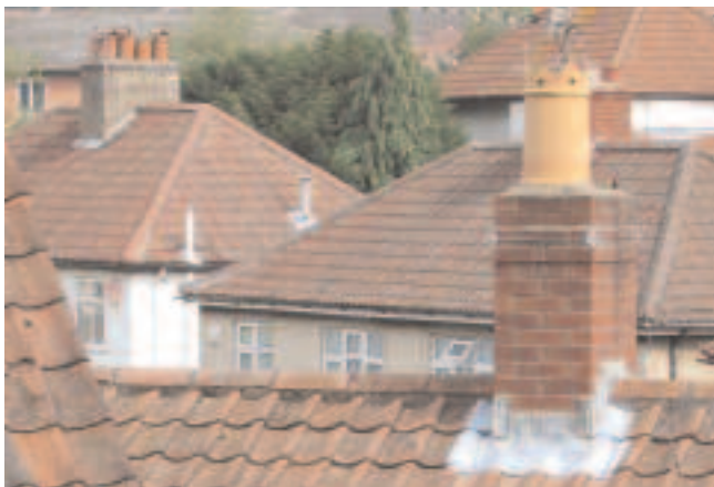
Alterations to prominent roofs needs careful consideration
