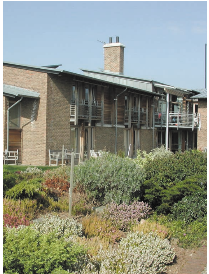
Well designed recent social housing at Bengough House, Crow Lane, Henbury
