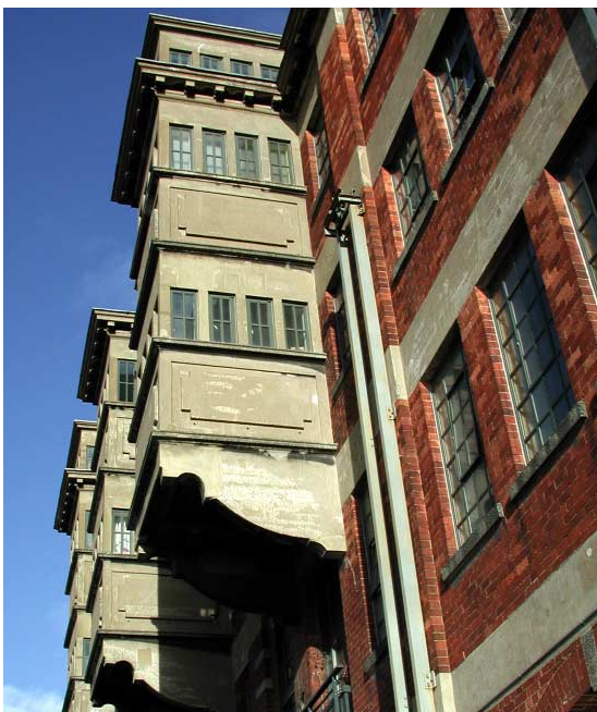
Conversion of the former WCA warehouse building, Redcliffe.
