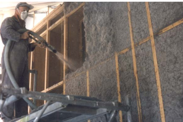
Warmcell insulation made from recycled newspapers to insulate walls.
