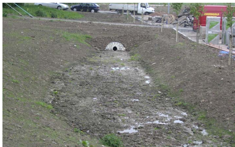
Sustainable drainage at Henbury School.
