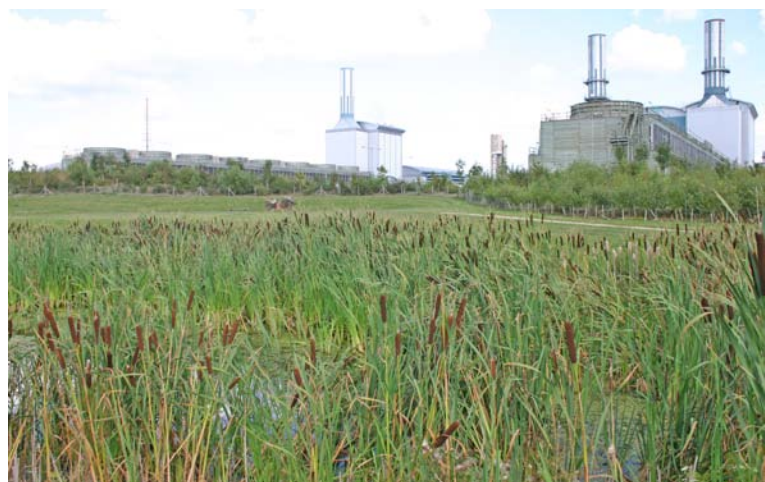
A wildlife pond incorporated into the design of a new amenity area around Seabank Power Station at Avonmouth.
