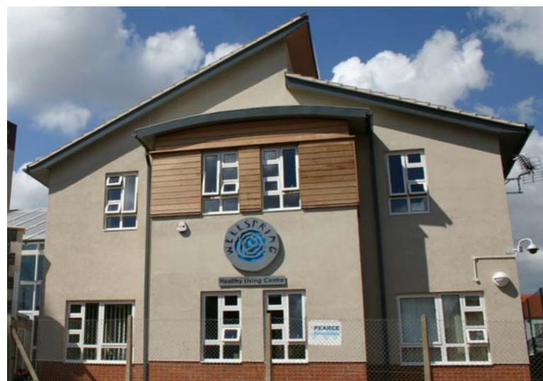
Wellspring Healthy Living Centre in Barton Hill has been designed to be naturally cool in summer and warm in winter.
