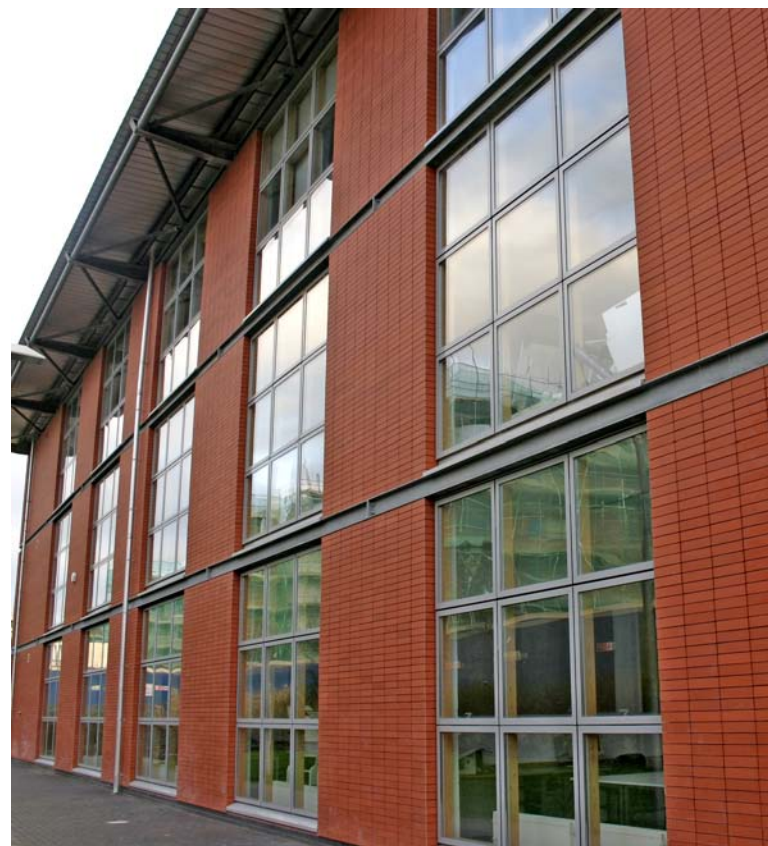
Maximising solar gain in winter with large glazed areas, and a roof overhang to provide shade in summer - the architecture studio at UWE.
