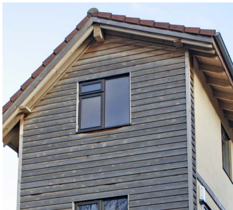
Use of sustainably sourced timbers at Ashley Vale self-build site.
