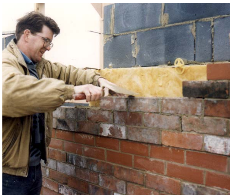
Re-used bricks were combined with new to build the lower walls of the Ecohome at CREATE.
