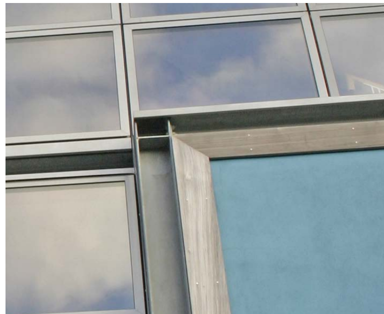
Interesting use of materials from glazing to straw bale panels at the UWE architecture studio.
