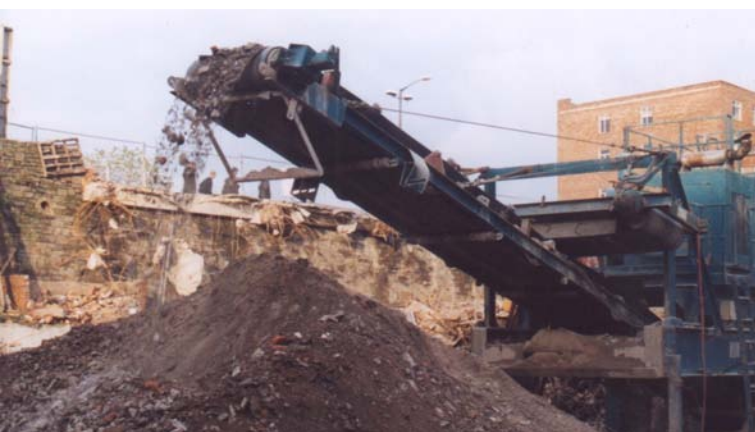
Grinding up demolition waste for re-use.
