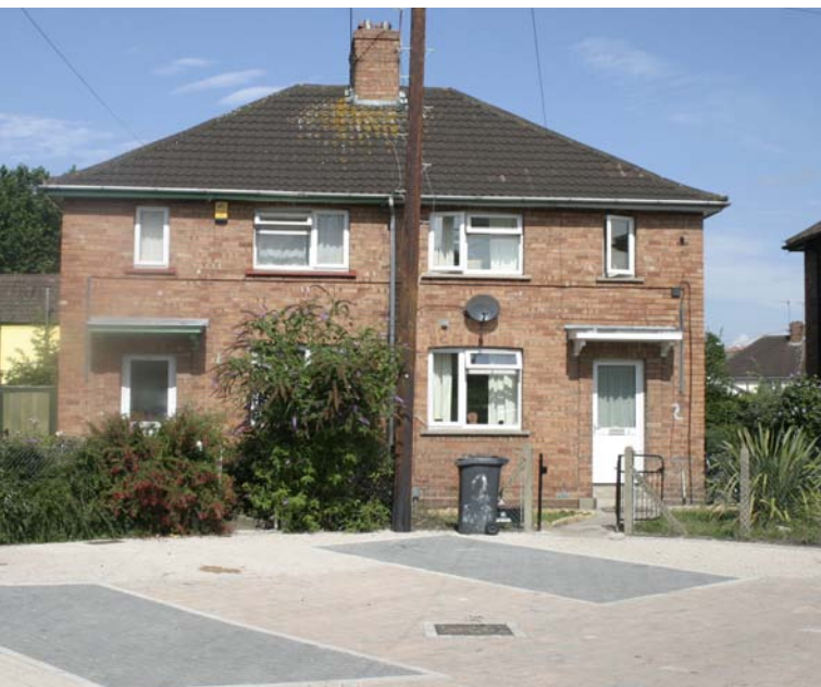
Permeable paving in the Dings homezone.
