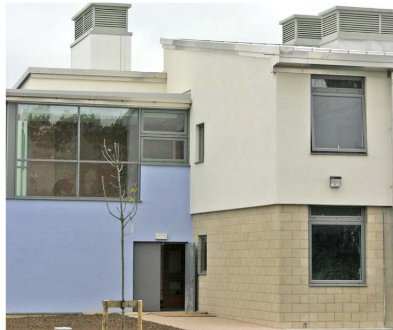
Natural ventilation used at the new Henbury School.
