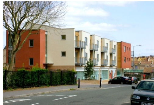
1. Barton Hill, Bristol Achieved Building for Life Silver Standards, 2010
