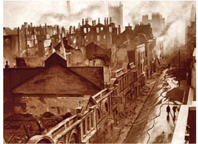
Figure 8: Bomb damage to Union Street, looking south. The redevelopment of this area resulted in Broadmead
