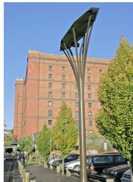
Trial of a solar powered street light outside the CREATE Centre
