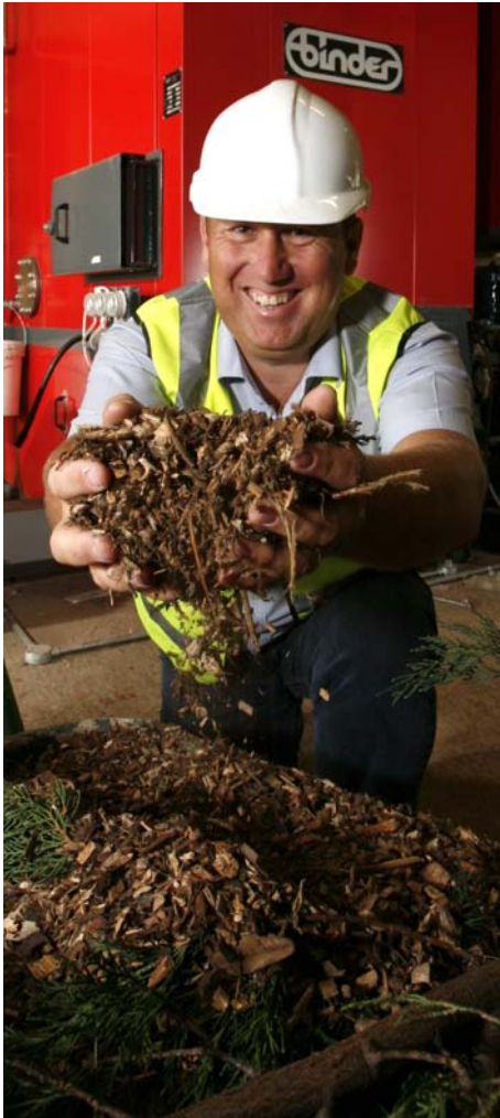
Award-winning biomass boiler at Blaise
