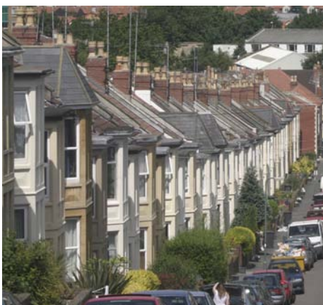
Energy efficiency measures in buildings can achieve significant CO 2 reductions
