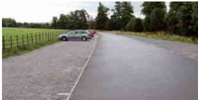
The new Church Lodge car park
