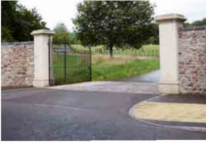
The new Ashton Road entrance
