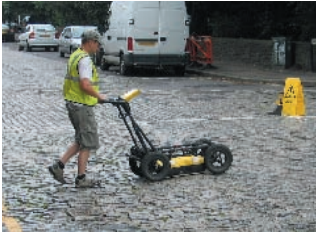
Ground Penetrating Radar survey in progress
