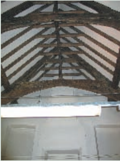
Medieval roof in Bakers Hall, Quakers Friars
