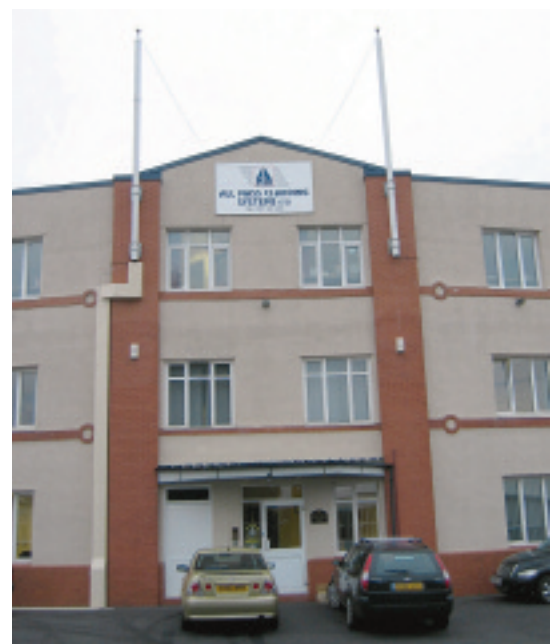
Flagpoles at Cater House - one concealing three antennae
