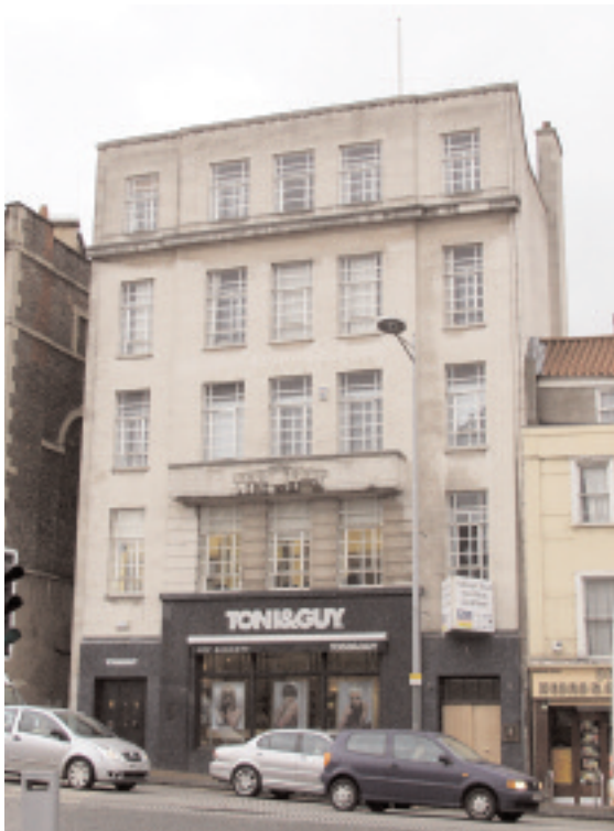
Flagpole replacing antennae, 1-2 St Augustines Parade
