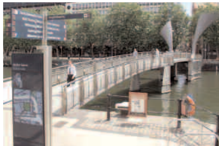
The construction of Pero's Bridge was secured through the use of planning obligations
