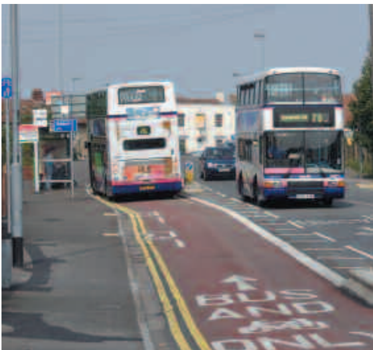
Showcase bus route - Parson Street contra-flow bus lane funded through Planning Obligations
