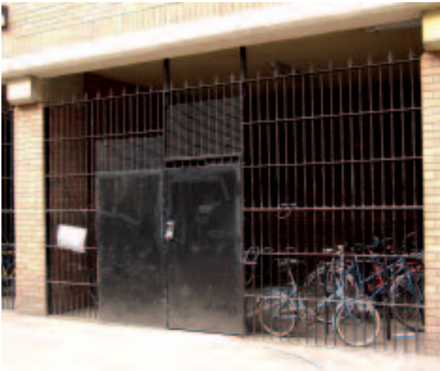
(A) Provision should be made to independently lock cycles within the compound - Sheffield stands make the best use of space and offer the highest security.
