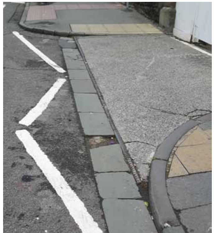
Fig.12 Pennant and iron curb at former site threshold on Lower Maudlin Street
