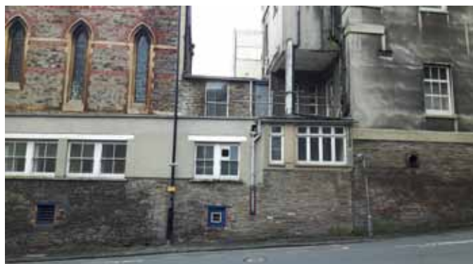
Fig.10 Former line of Earl Street blocked by Pennant sandstone wall (paler stonework) erected in 1825
