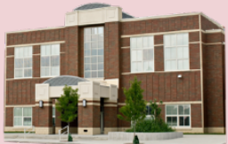
Ashton Gate Primary School
