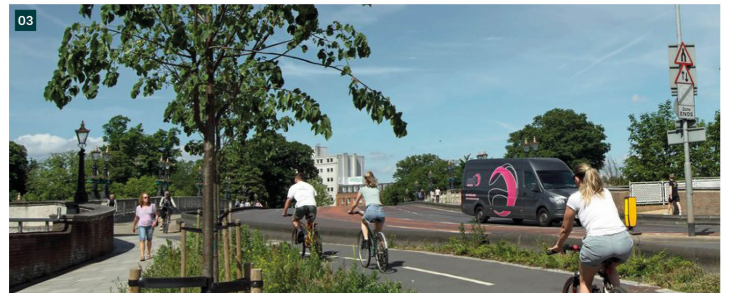
Fig 07.32 Aspirational street network precedents demonstrating good modal balance, green infrastructure provision and pedestrian safety
