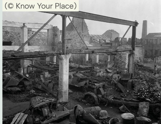
War damage to 72-74 Feeder Road.
