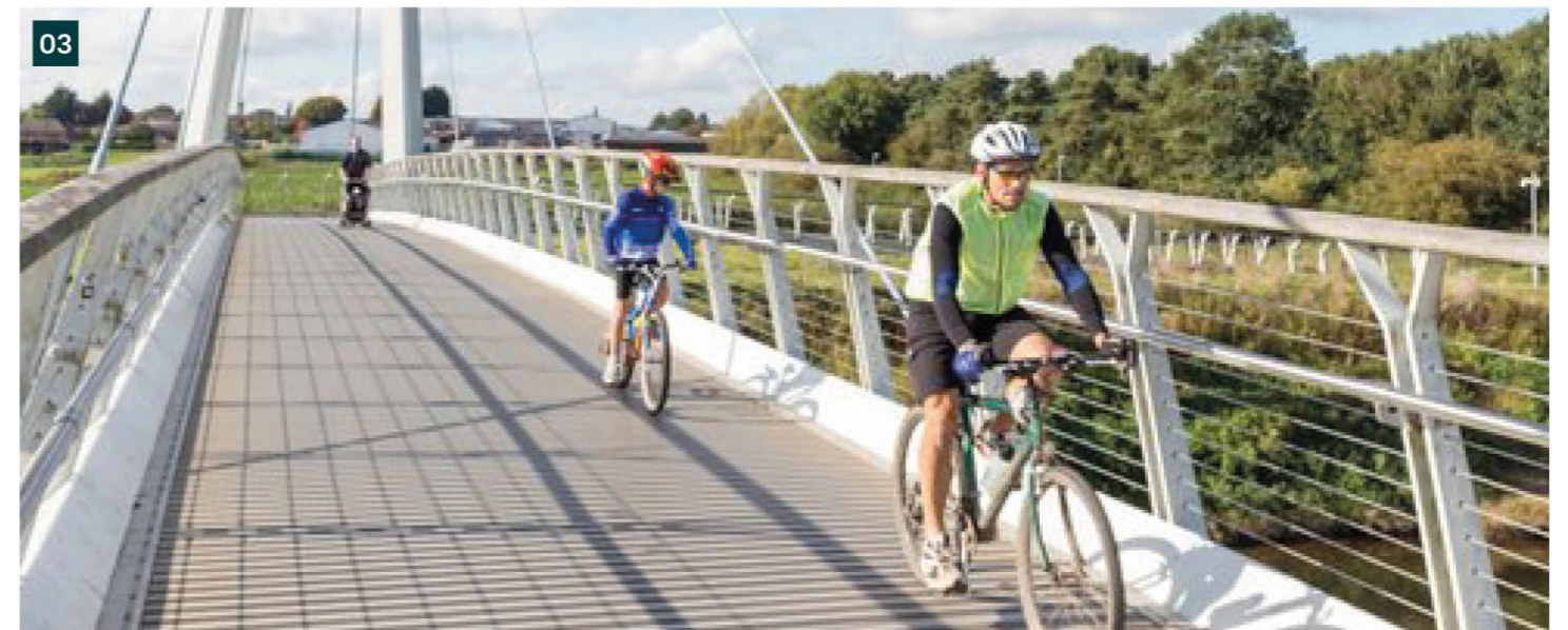
Fig 07.07 Aspirational cycling infrastructure provision
