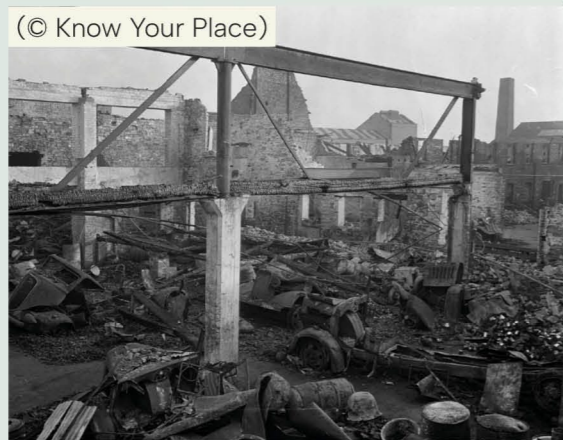
War damage to 72-74 Feeder Road.
