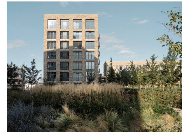
Image 29 – Luscious planted gardens can be delivered at podium level above ground floor shops. © Tim Crocker
