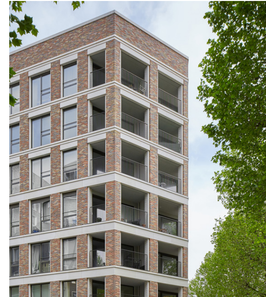
Image 35 - Recessed balconies can be highly functional, providing a good balance of daylight, privacy and shelter. © Tim Crocker
