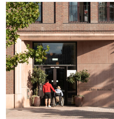
Image 20 - The entrance design is clearly marked through a change in material palette and scale, whilst the recessed building line provides shelter and space for planting, adding to a sense of personalisation. © Tim Crocker
