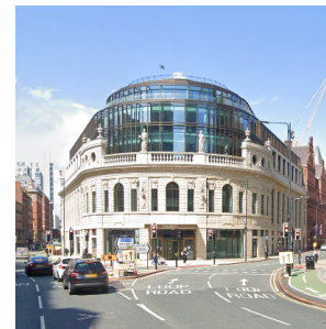
Image 10 - A change of materials and fenestration are used here, whilst the structural facade proportions are reflected through the horizontal articulation of upper floors. © Google Maps.
