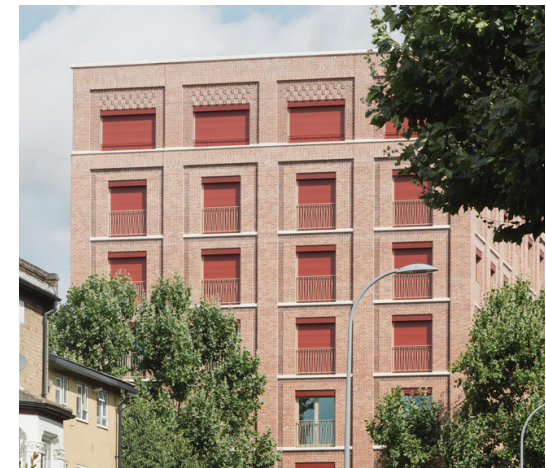
Image 38 – Reduced window area on upper levels takes advantage of less overshadowing, whilst external movable shutters are well integrated into the facade design. © Tim Crocker
