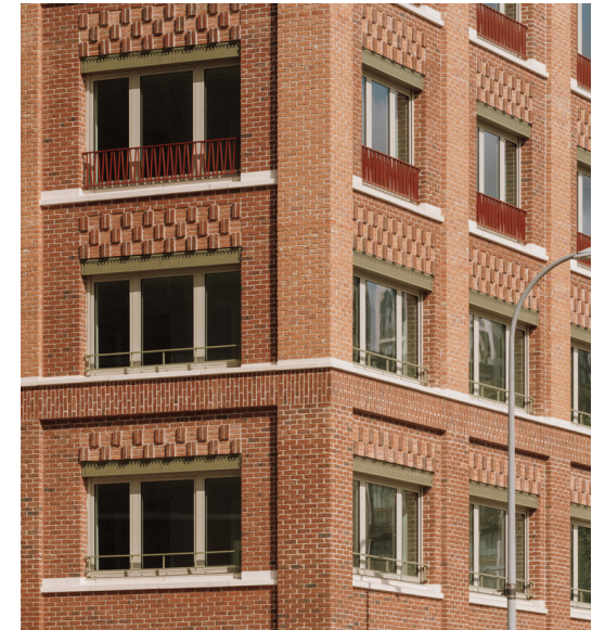
Image 37 – Stepped reveals or textured panels can improve the appearance of horizontal window proportions. © Tim Crocker
