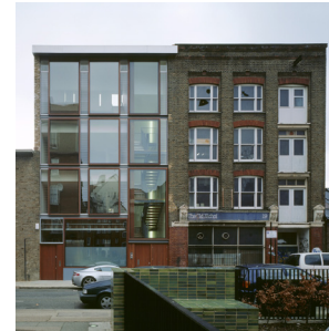
Image 6 - The facade proportions of the historical building are expressed through contemporary fenestration and material choices. © Helene Binet.
