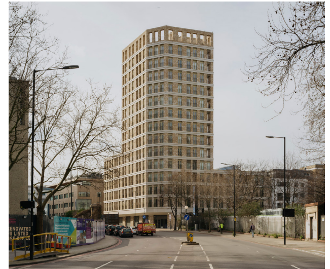
Image 26 - Height transitions in scale, stepping down from the corner to meet the building height datum of adjacent buildings. © Tim Crocker
