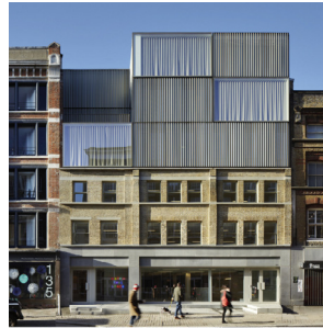
Image 5 - Key proportions are reflected in the vertical extension, with innovative use of new materials and approach to fenestration. © Jack Hobhouse.
