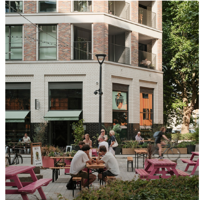
Image 21 - Chamfering the building line creates pocket space for public realm and facing into the corner with active frontage creates natural surveillance. © Tim Crocker
