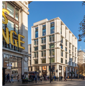
Image 9 - New development takes material, massing and proportion cues from the heritage building, whilst increased use of glazing distinguishes it as clearly contemporary. © Nick Kane.
