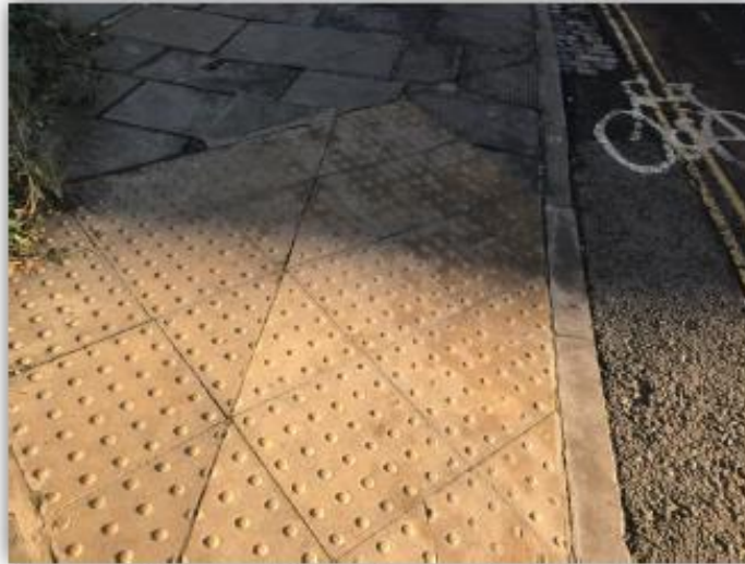
Image of the tactile pavign at the Woodland Road junction.
