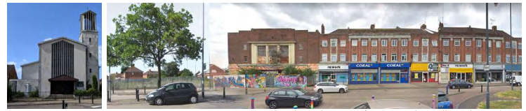
View from the East - frontages along Filwood Broadway
