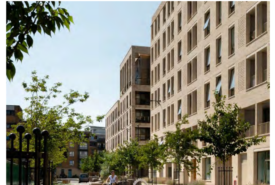
Precedent: Medium rise residential development in the King's Crescent Estate, London. New street trees line the new frontage.
