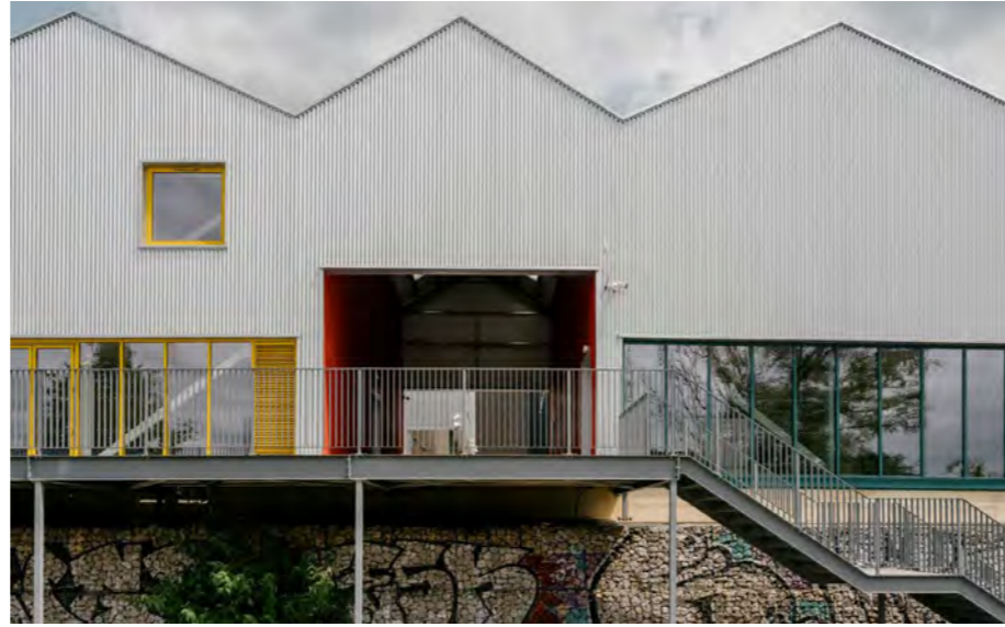
Hackney Bridge, London. Designed as a meanwhile use for an interim period of around 15 years, providing 'incubator' space for local creative businesses.
