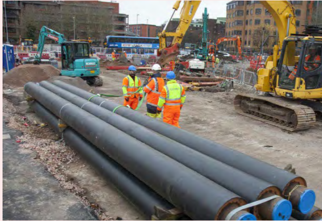
Installation of Redcliffe heat network
