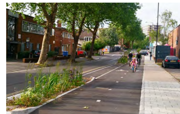
Existing Whitehouse Street cycle track.
