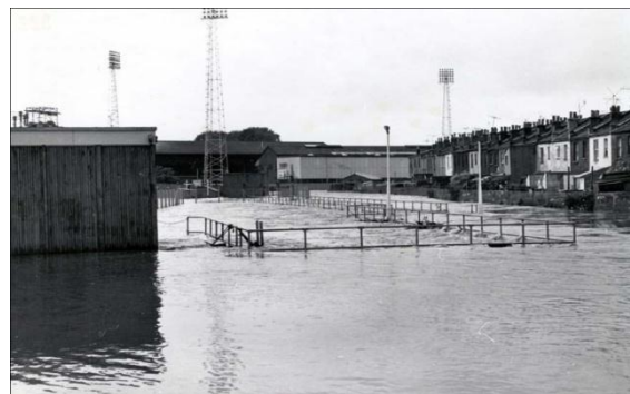
Plate 2 Flooding in Eastville 1968 (Source: BCC)
