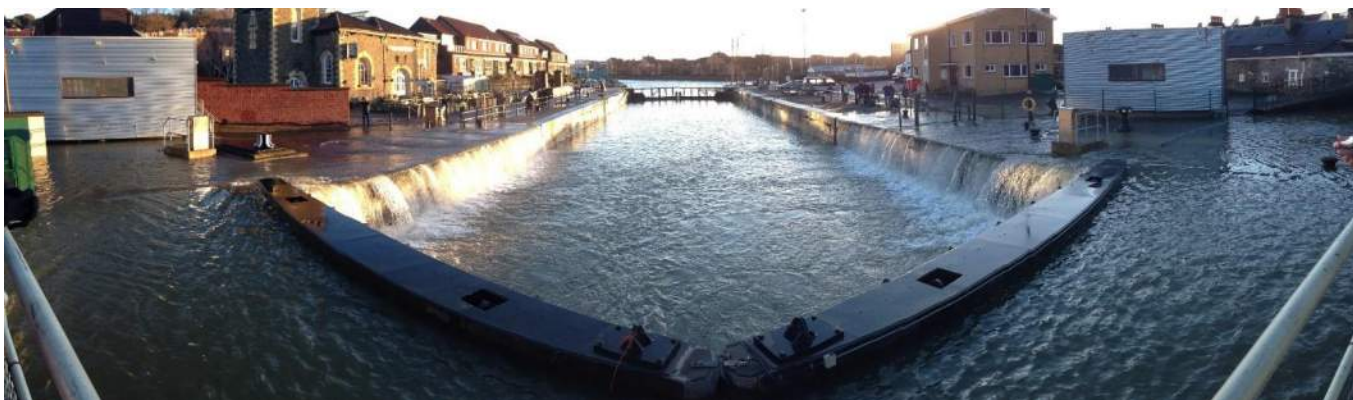
Figure 1: January 2014 tidal surge inundating the A4 Portway in the Avon Gorge (top), Cattlemarket Road (left) and Clarence Road (right), and outflanking tidal flood gates at Junction Lock into the Floating Harbour (bottom).
