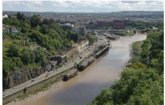
Figure 8 View of Entrance Lock from downstream
