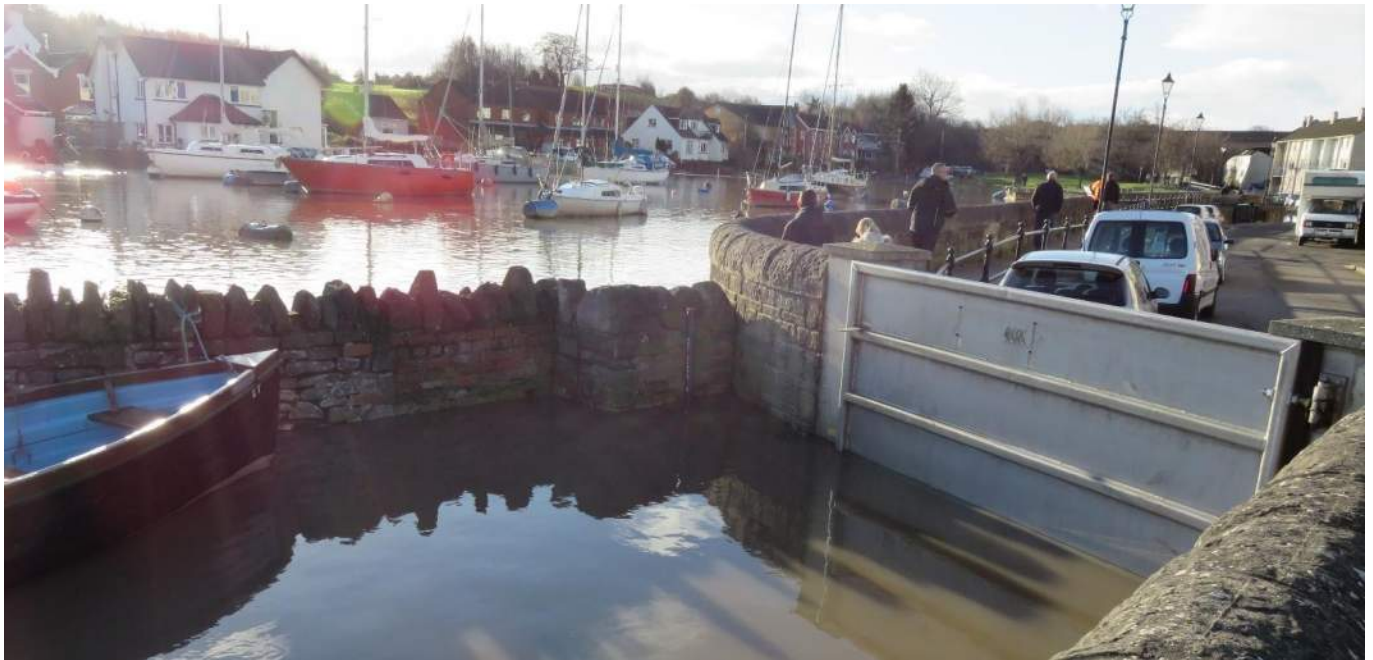
Figure 25: Existing flood defences in operation at Pill
