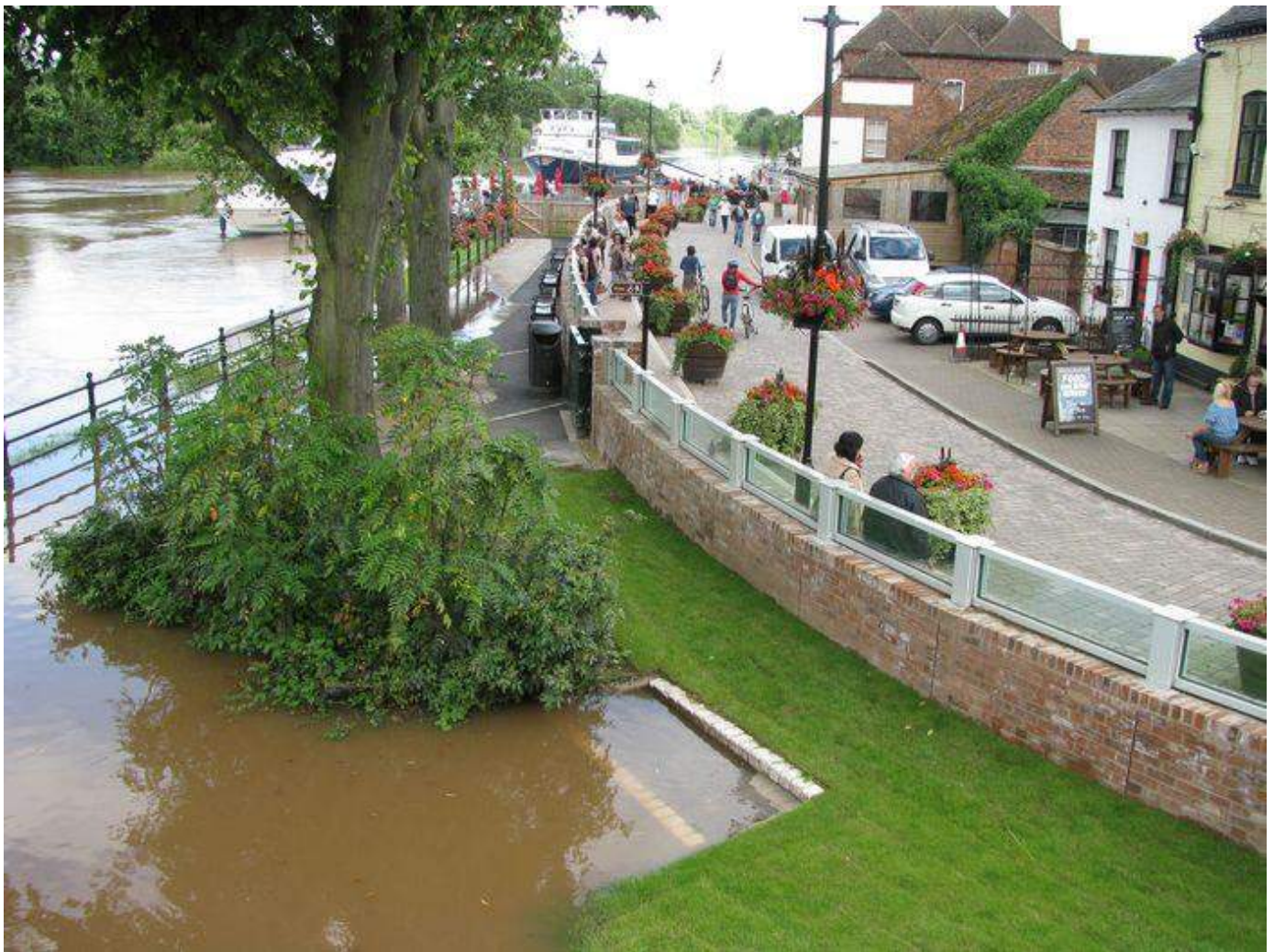
Figure 36: Flood defences including glass panels installed in Upton upon Severn
