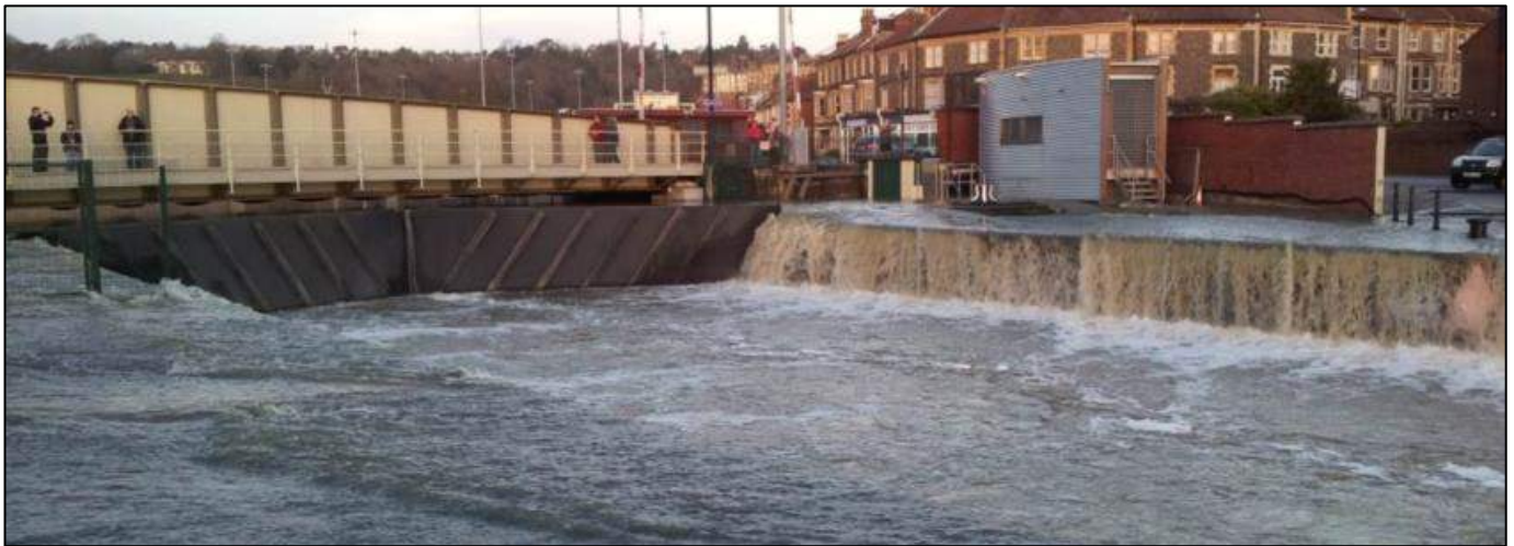
Figure 19: Water shown overtopping the Junction Lock stop gates into the Floating Harbour
