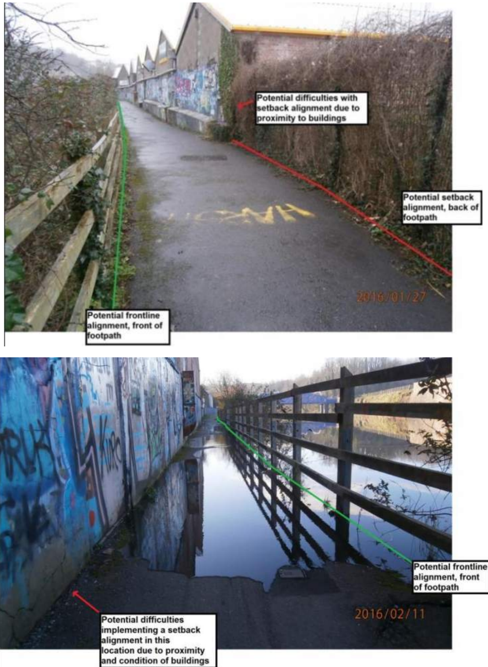
Figure 3: Showing typical constrained section. Note comments are from AECOM's preferred option development report
