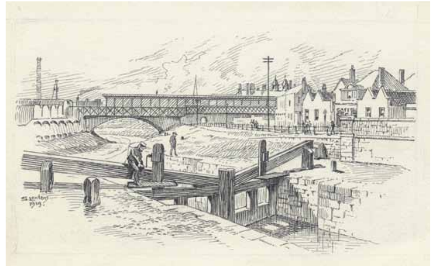
Fig 41 Early 20th century drawing by Samuel Loxton of Totterdown Lock, Bristol Archives, U1146
