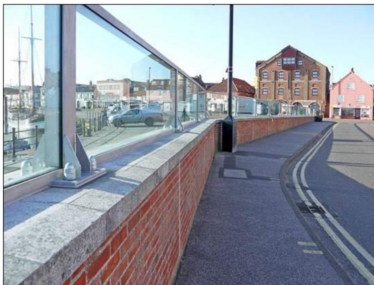
Figure 7: Example flood defence measures
