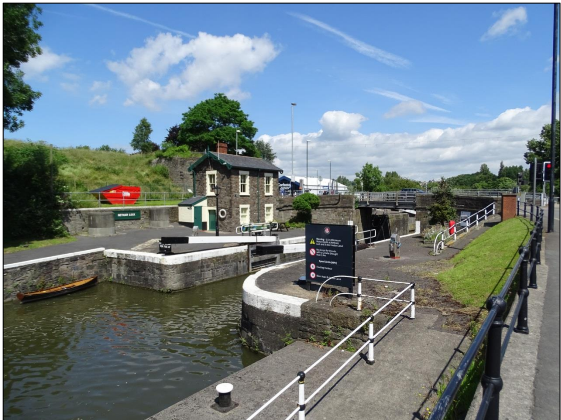
Figure 6. Lock gates at Netham (open position, looking upstream to the north-east)
