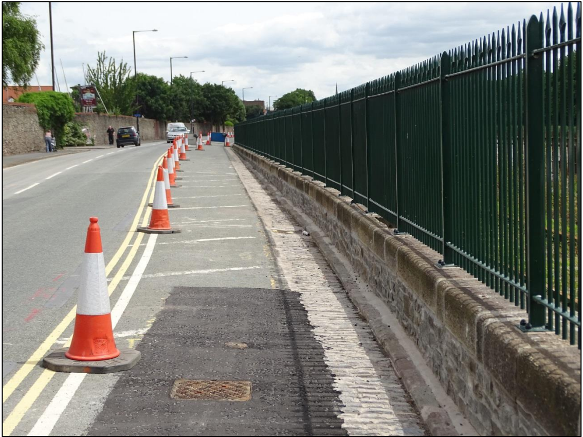
Figure 7. Newly constructed MetroBus flood wall (Cumberland Road)
