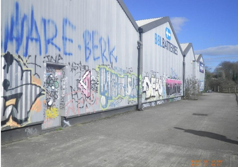
Figure 36 – Panel clad wall
