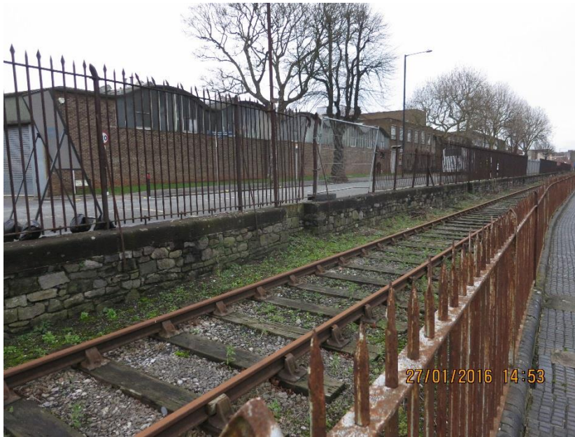
Figure 8 - Photo of the wall from the Chocolate path on the riverside The top of the wall extends above the road level by 150-250mm. Best estimate as to the condition of the wall is condition grade 3.
