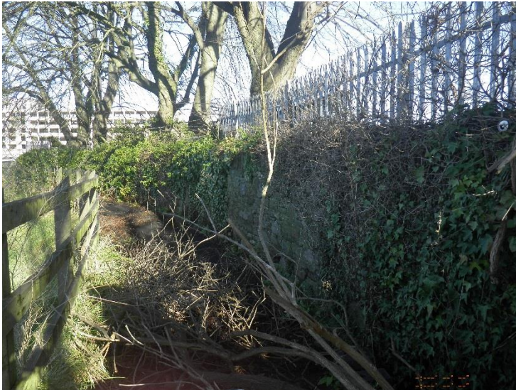
Figure 17 – Photo showing stone wall looking downstream.
