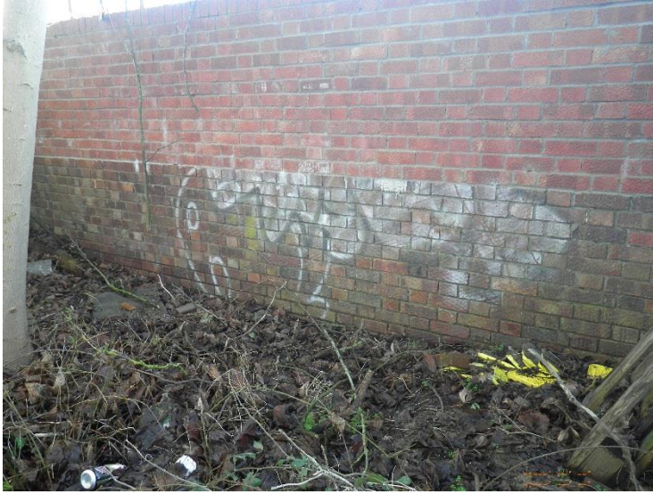
Figure 18 – Photo showing brick wall
