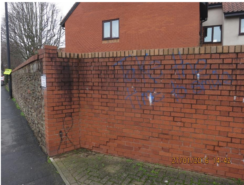
Figure 7 - Photo of the clay brick wall close to Vauxhall Bridge
