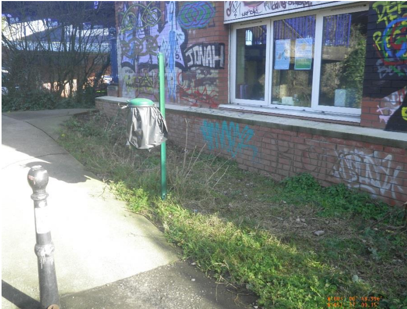
Figure 24 - Wall of RSPCA Bristol Dogs and Cats Home, adjacent to the flood defence asphalt ramp can be seen on the left
