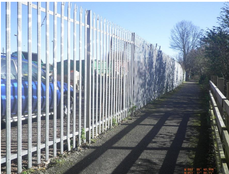
Figure 29 - Palisade fencing adjacent to Venture Tyres building
