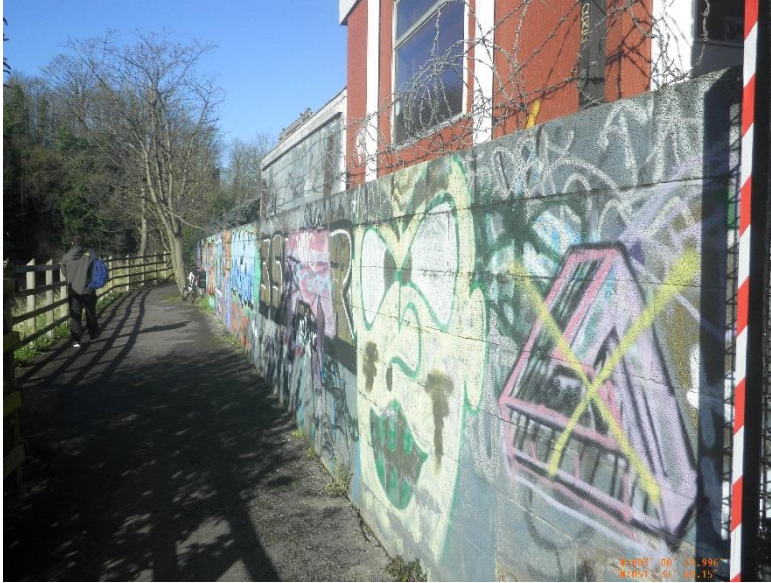
Figure 27 - Concrete block wall
