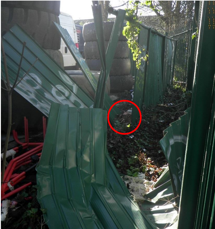
Figure 19 - The brick wall can be seen immediately behind the steel panels
