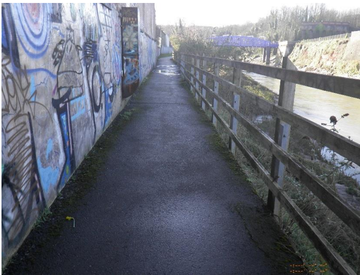
Figure 21 – Wall of building, looking upstream.
