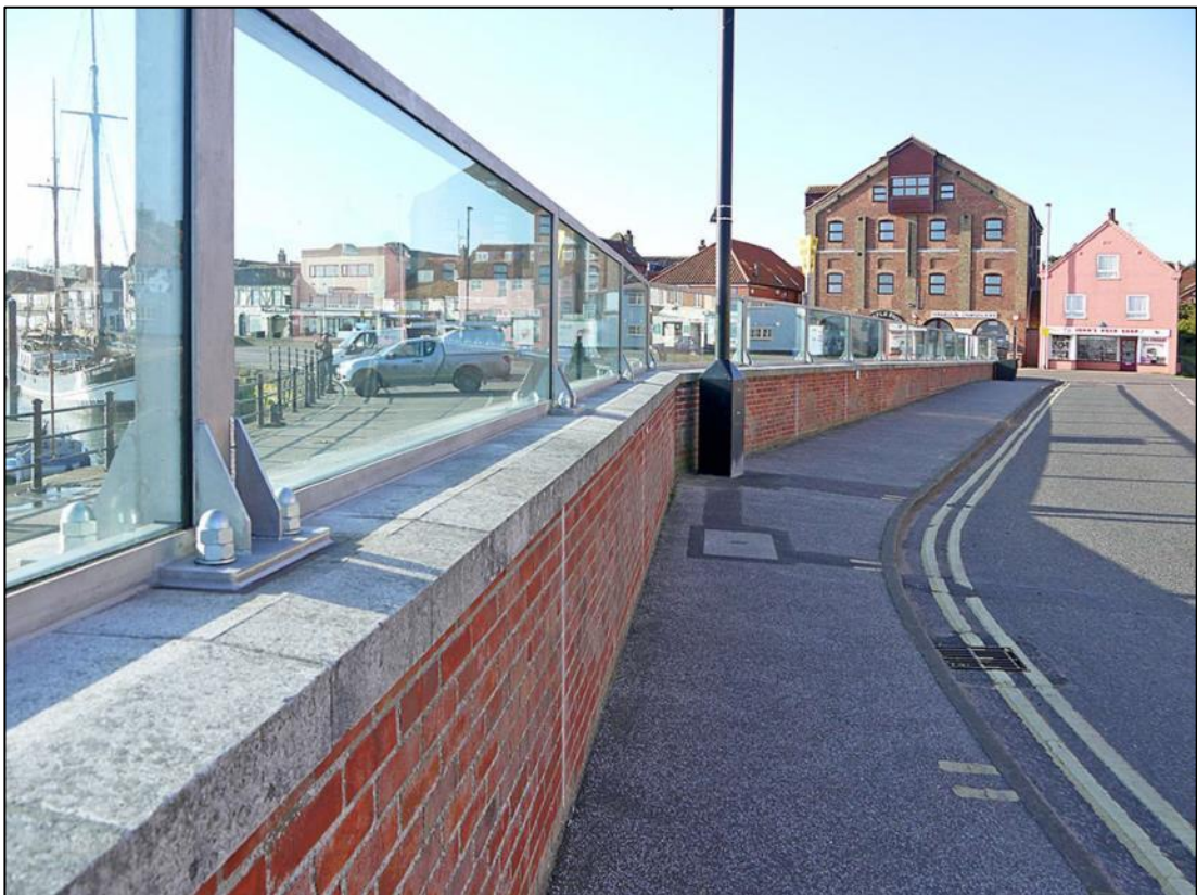
Figure 15 Example of a reinforced glass floodwall (image courtesy of Flood Control International. Available at www.floodcontrolinternational.com )
