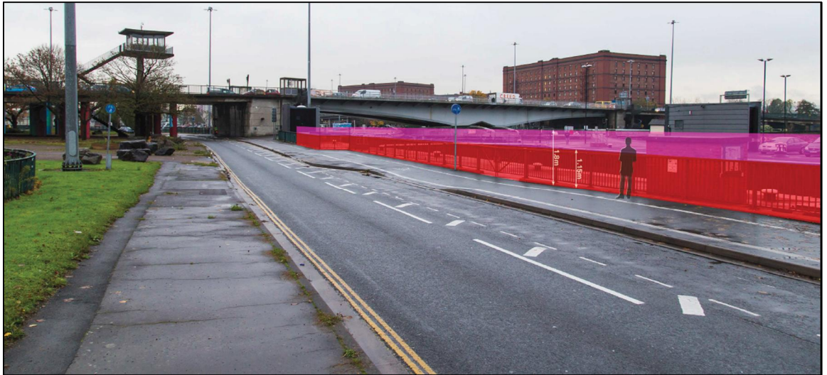
Figure 5 Landscape visualisation of the proposed defence at Entrance Lock (low defences shown in red, high defences in pink)
