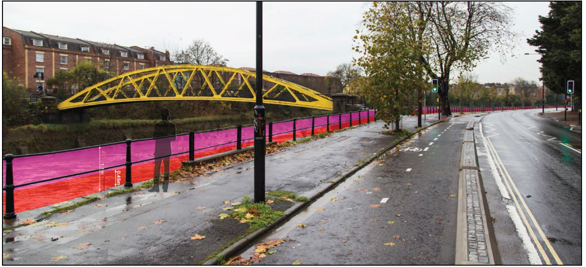
Figure 12 Landscape visualisation of the proposed defence at Clarence Road (low defence in red, high defence in pink)
