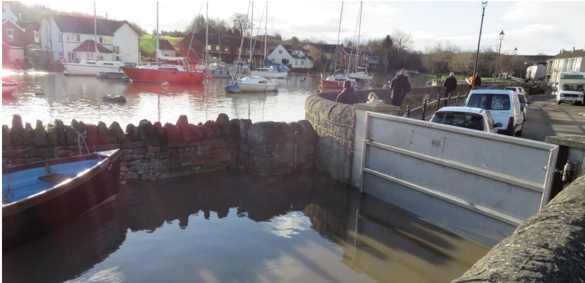
Figure 20 – Existing flood defences in operation at Pill
