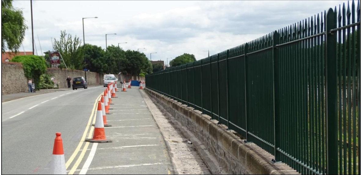
Figure 17 - The MetroBus flood wall on Cumberland Road
