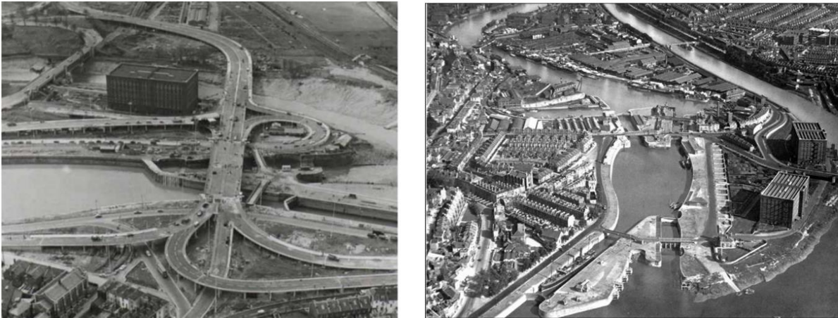
Figure 16 - Construction of Junction Lock, 1964 (left) and Brunel Harbour, 1929 (right)
