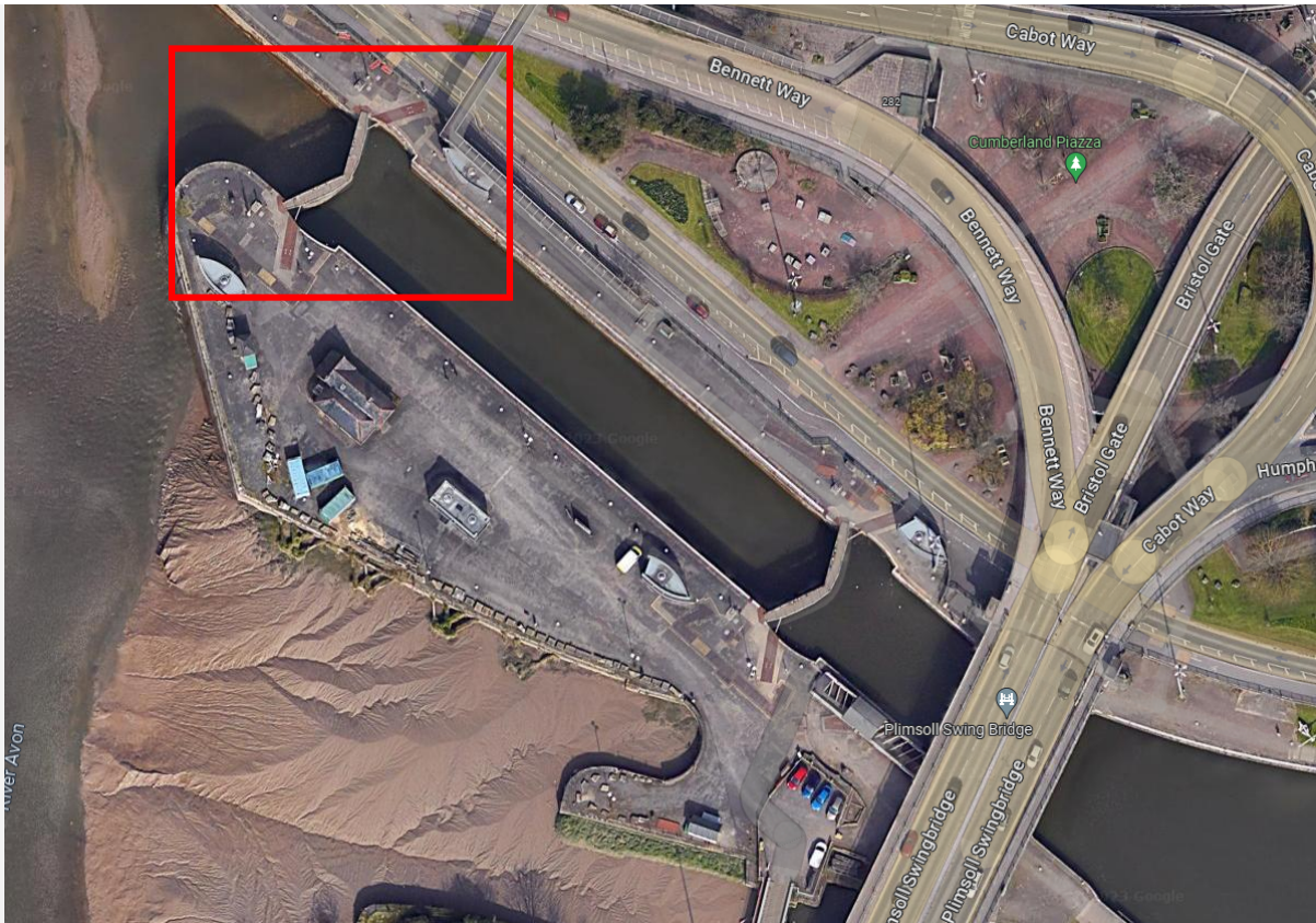
Fig 1 : Bristol harbour entrance (outer) lock gates
