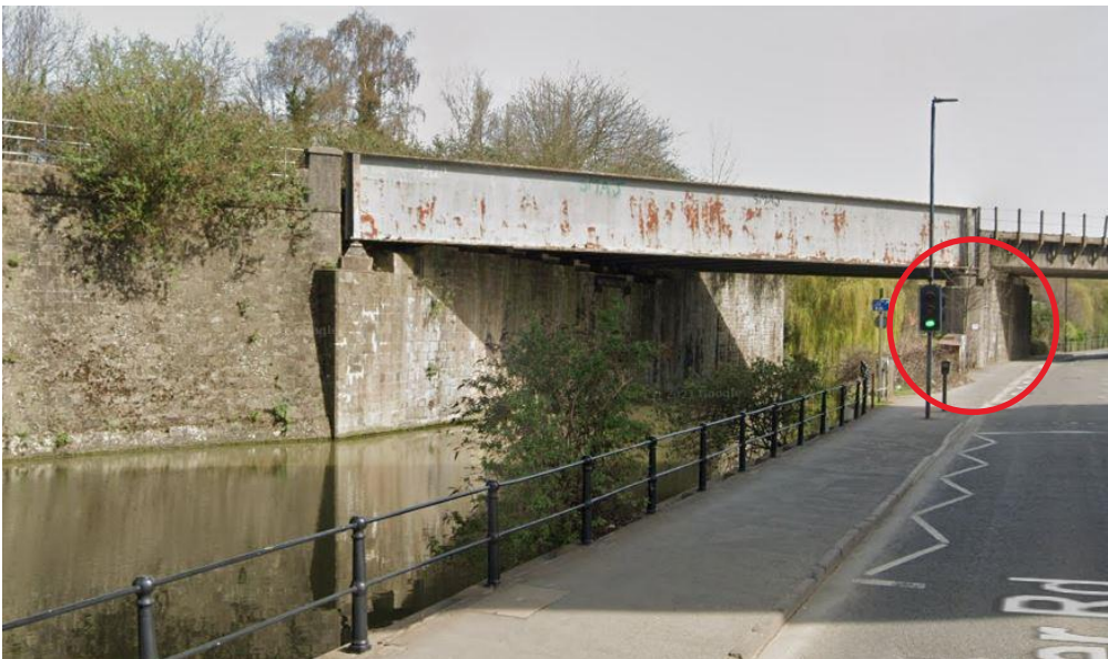
Figure 3: Rail bridge pier at 360810,172600. © Google.
