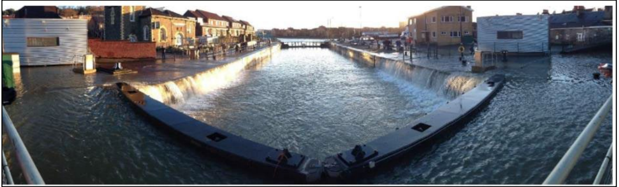
Picture 2: Flood flows bypassing the lock gates.
