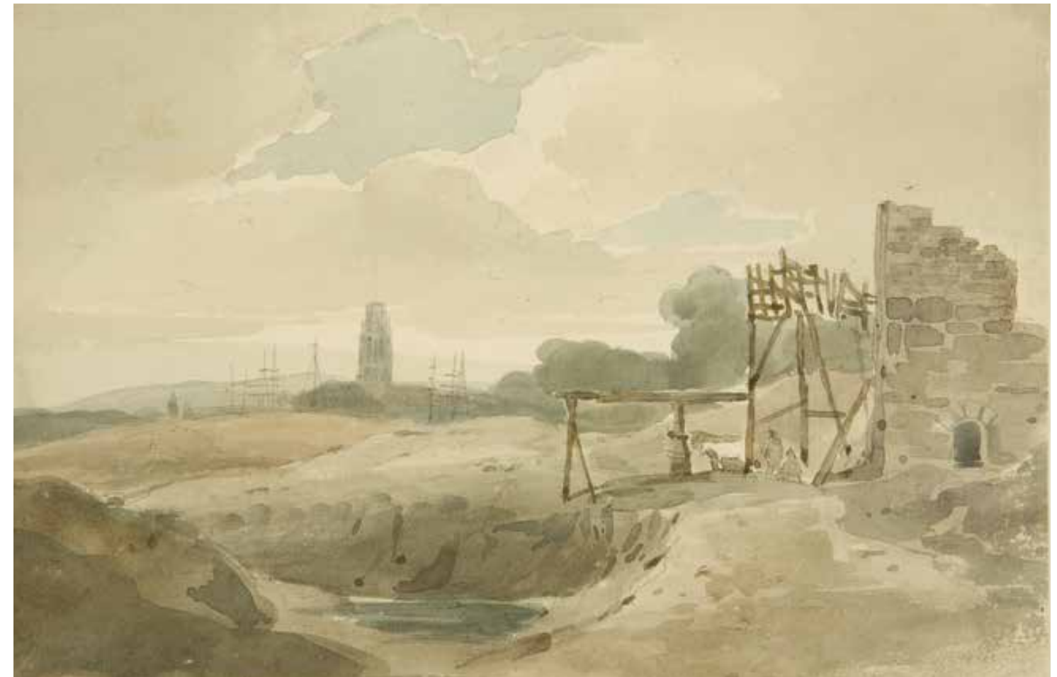
Fig 57 The only known image of part of the New Cut construction infrastructure. This painting by Rev. John Eagles produced in the early 1820s shows the derelict remains of an engine house for a fire [steam] engine, used between the Ropewalk at Wapping and Clift House during the excavation of the New Cut 1804 to 1809, Bristol City Museum and Art Gallery, M2958
