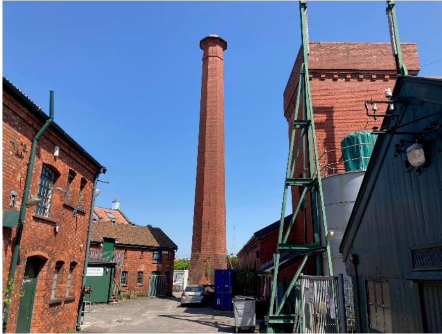
Photograph 5:Chimney, Underfall Yard
