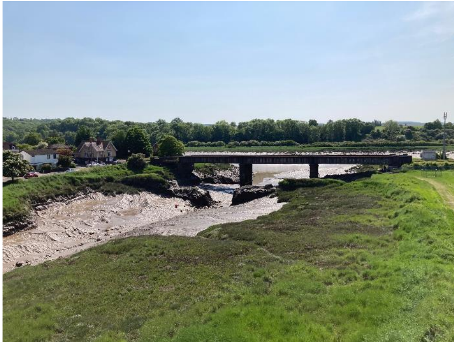
Photograph 3: Railway bridge and historic dock walls at Sea Mills, viewed from Portway Bridge
