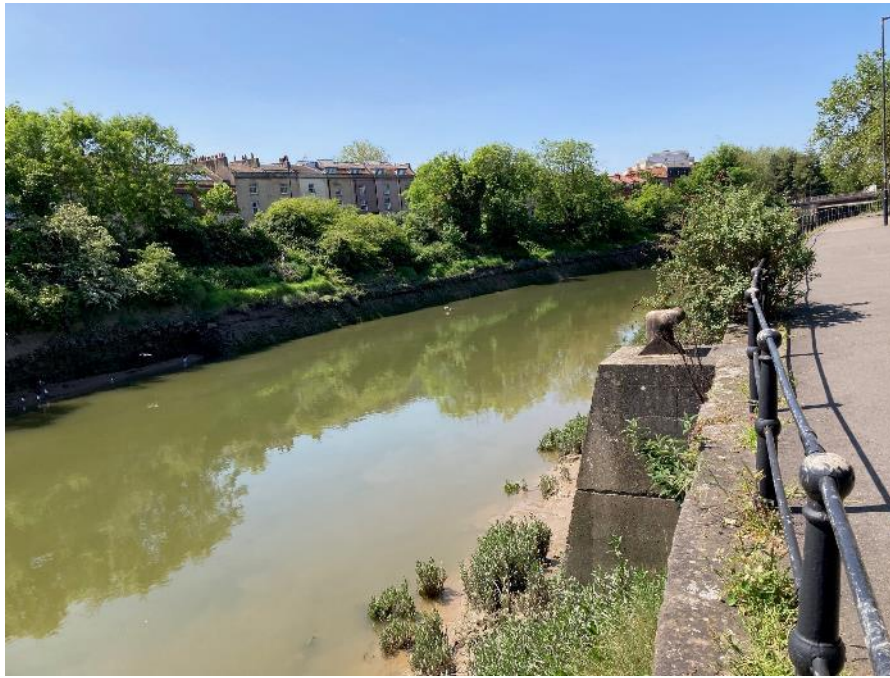
Photograph 8: The New Cut from Clarence Road, looking west
