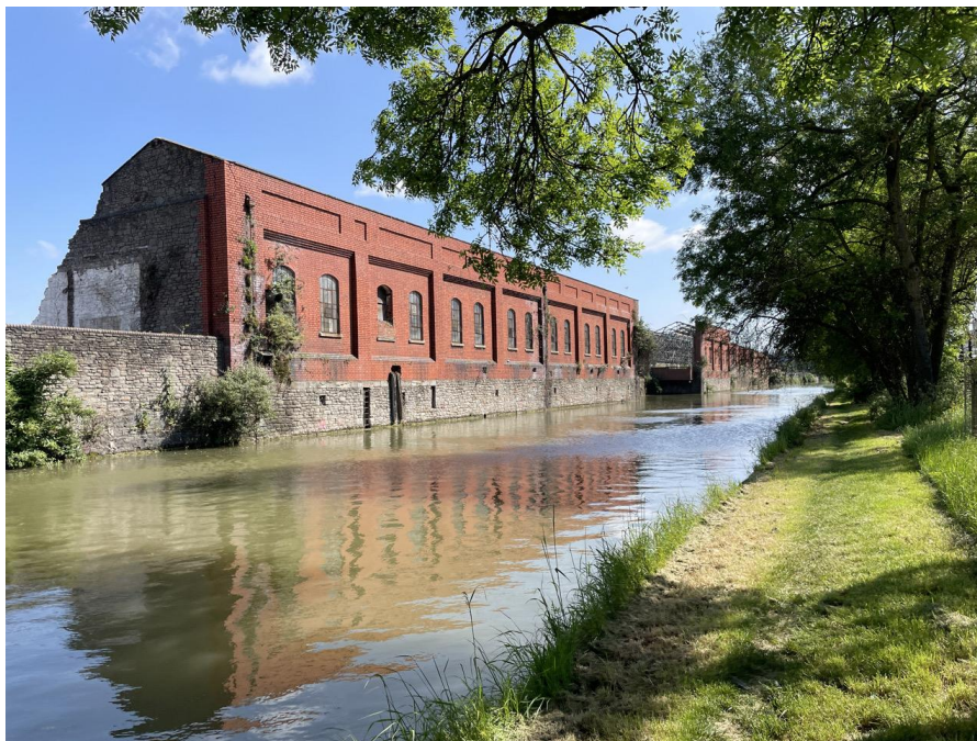
Photograph 10: St Vincent's Works, viewed from the south side of the Feeder
