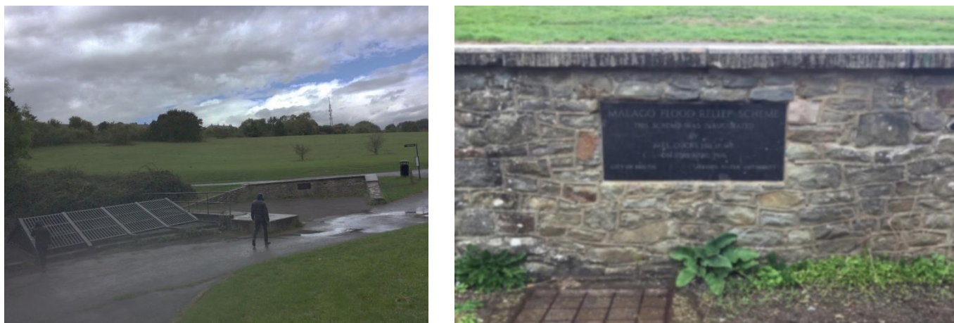
Figure 20 - The Malago Flood Relief Scheme
