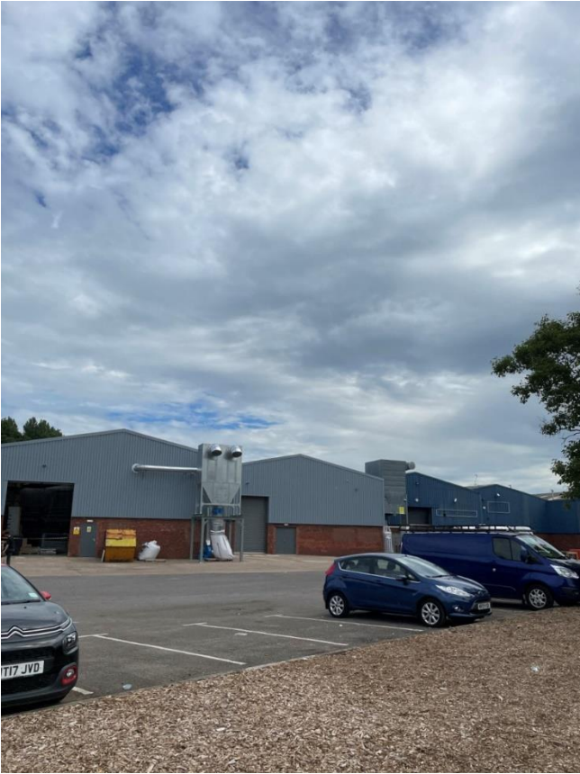
Photograph 6. Industrial estate at Netham.
