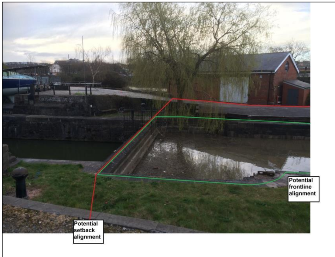
Figure 18 Potential defence alignments at Bathurst Basin Dam
