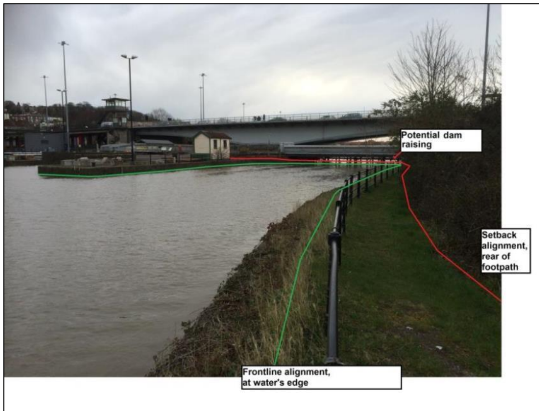
Figure 28 Potential defence alignments at Brunel Dam. Photograph looking east
