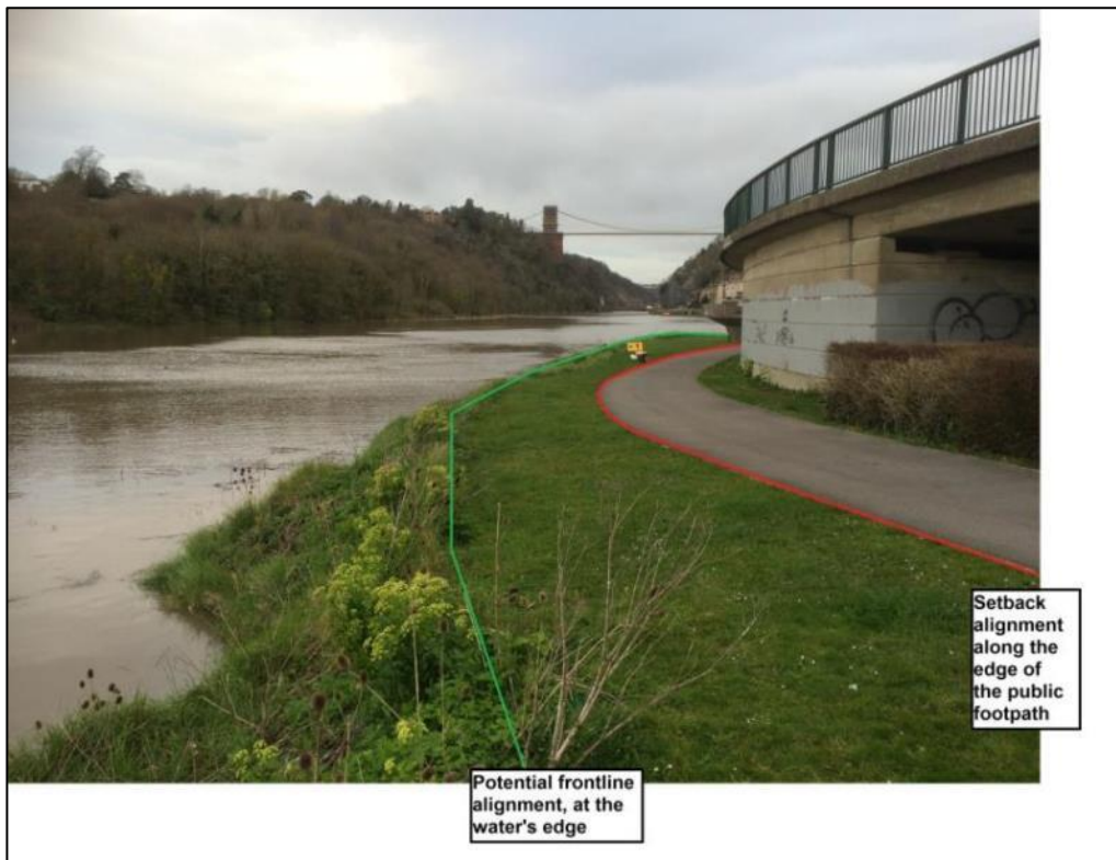
Figure 26 Potential defence alignments along the north bank of the New Cut, immediately to the west of Brunel Way road bridge. Photograph looking west towards Clifton Suspension Bridge.
