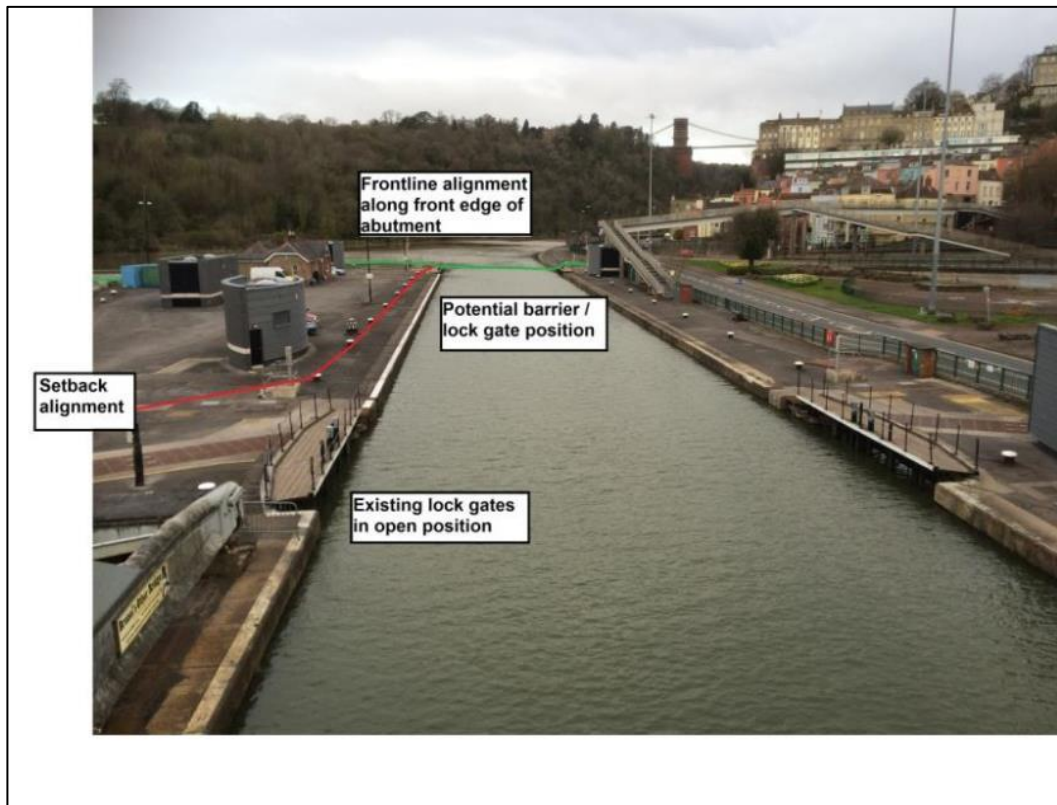
Figure 29 Potential defence alignments at Entrance Lock at entrance to Cumberland Basin. A potential lock gate position is also shown. Photograph looking west towards Clifton Suspension Bridge
