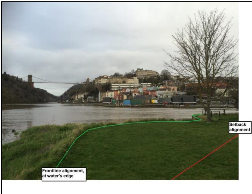
Figure 27 Potential defence alignments at the headland between the north bank of the New Cut and the southern entrance to Cumberland Basin. Photograph looking west towards Clifton Suspension Bridge
