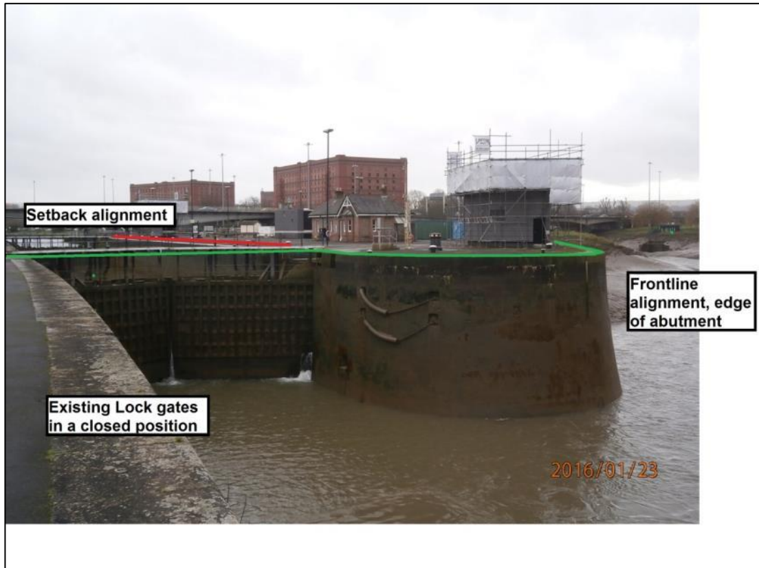
Figure 30 Potential defence alignments at Entrance Lock at the entrance to Cumberland Basin. The existing lock gates are shown in a closed position. Photograph looking east.
