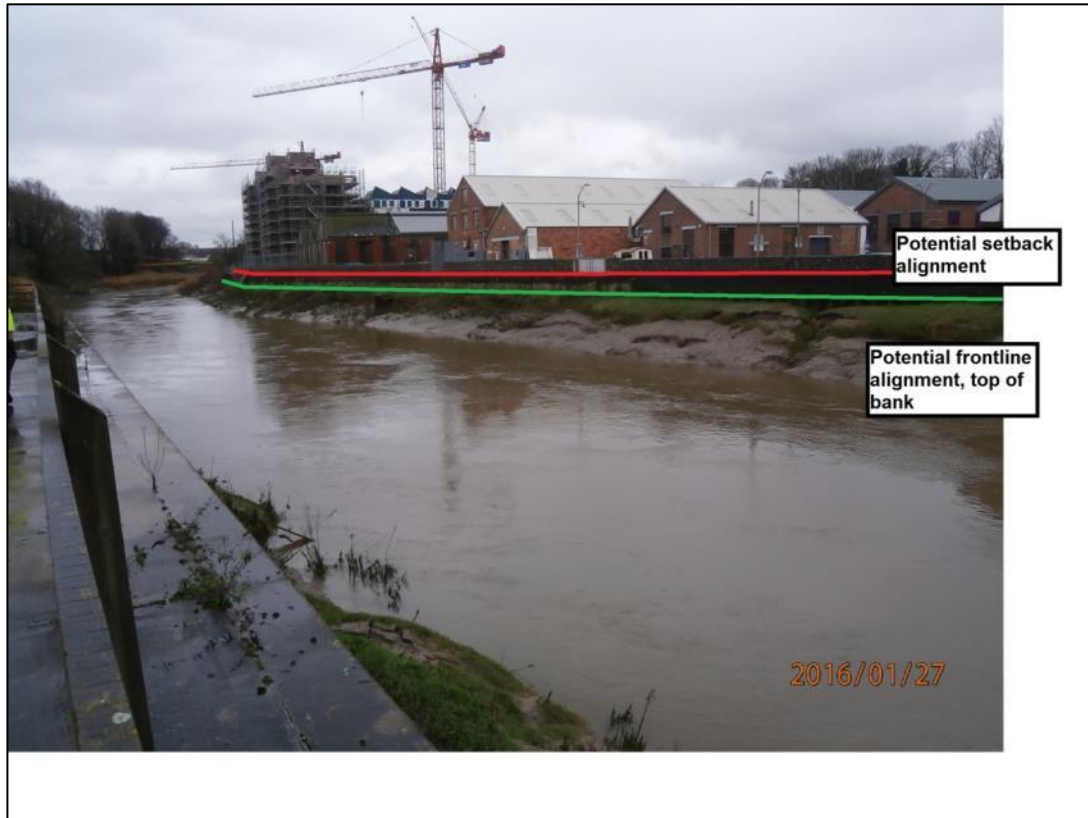
Figure 25 Potential defence alignments at Bath Road, photograph looking south east towards the frontage from the North bank of the New Cut
