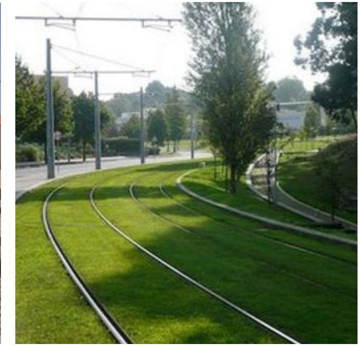
Metro do Porto has achieved careful integration of rails with hard and soft landscaping.
