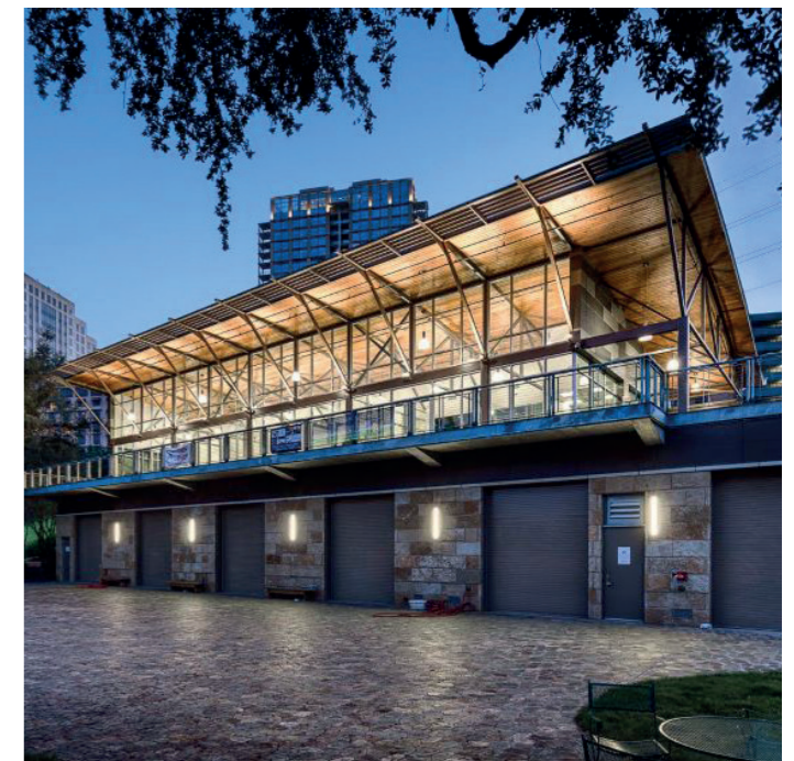
Waller Creek Boathouse, Austin, combines storage and technical spaces with office and leisure.
