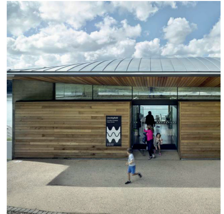
The Welsh Water Centre at Llandegfedd (2015) by Hall + Bednarczyk.
