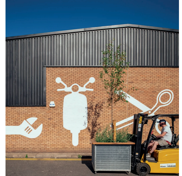
Above and Top Left Lockwood Way by We Made That has boosted the social, public and economic potential of an existing industrial estate.
