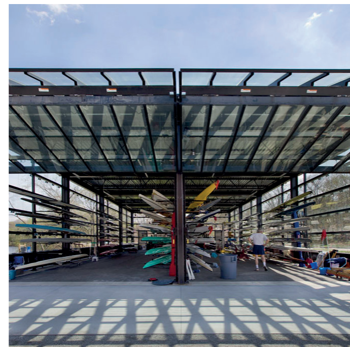
Community Rowing Boathouse boat storage, Boston, by Anmahian Winton Architects.
