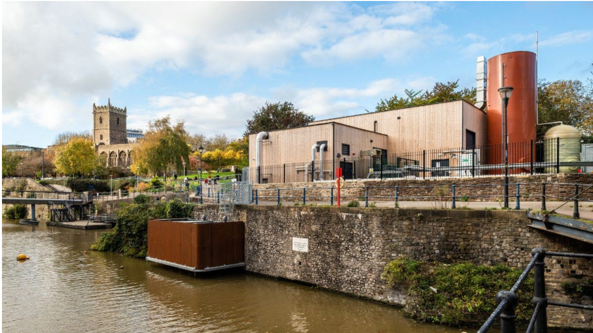
Figure 8: Energy centre in Castle Park, producing heat for the heat network using a large-scale water source heat pump
