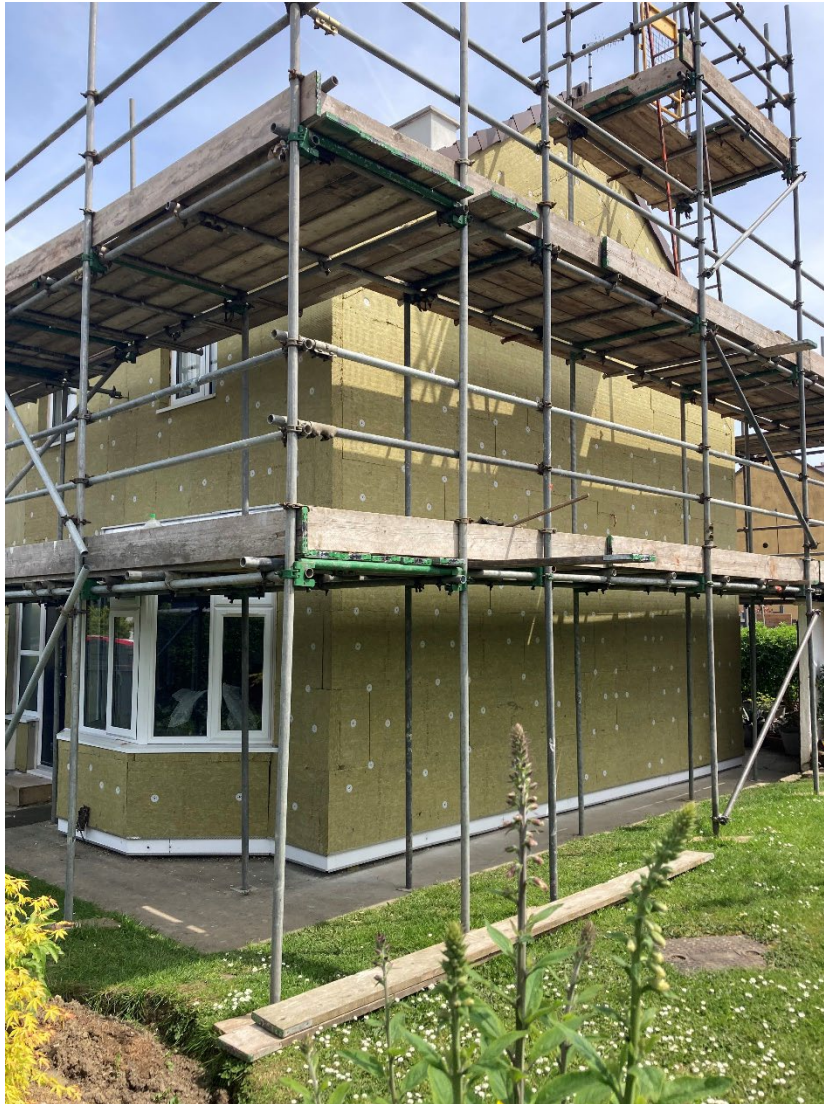
Figure 18: External wall insulation being installed on a Bristol City Council home.
