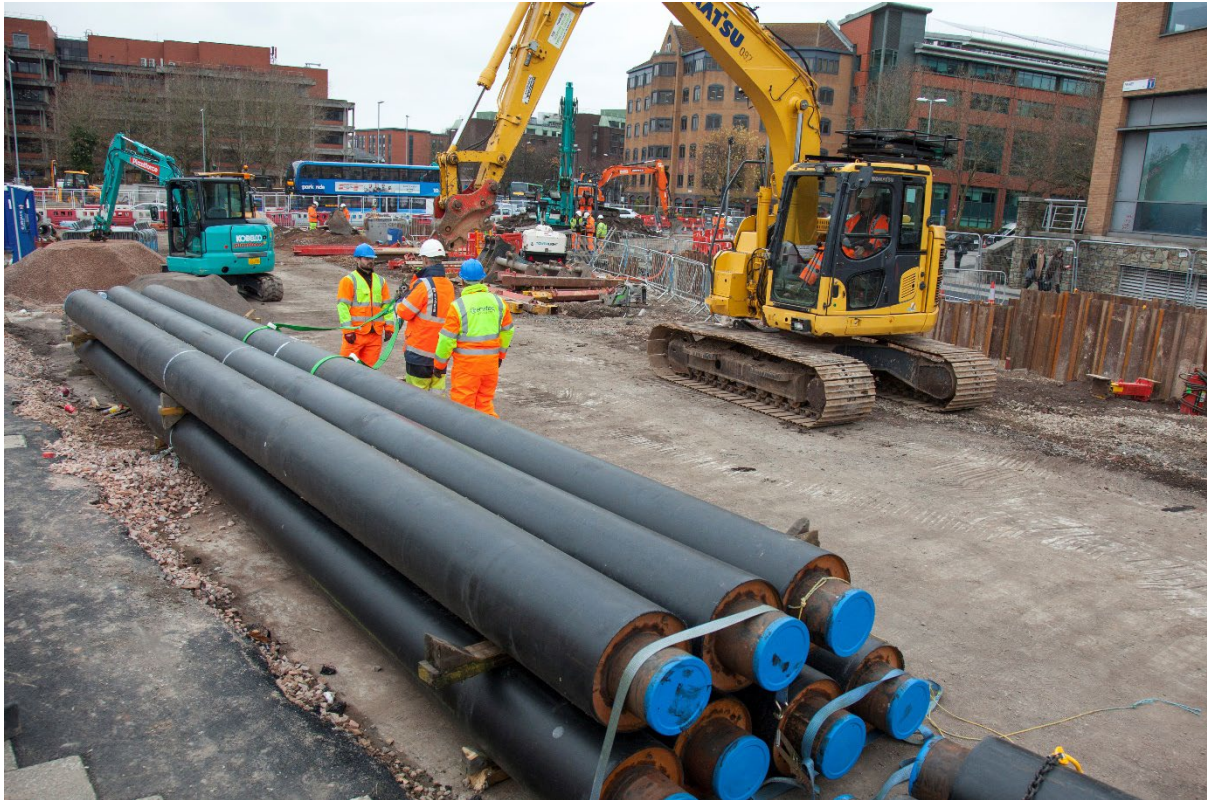
Figure 23: Heat network pipes being installed in Redcliffe.
