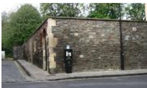
Figure 35: Pennant and limestone boundary wall, Wilson Street
