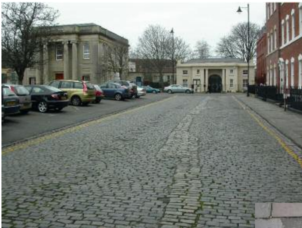
Figure 51 and 52: Whilst the east side of Brunswick Square retains its granite setts, reinstatement after placing utilities has been poor, creating an uneven surface.
