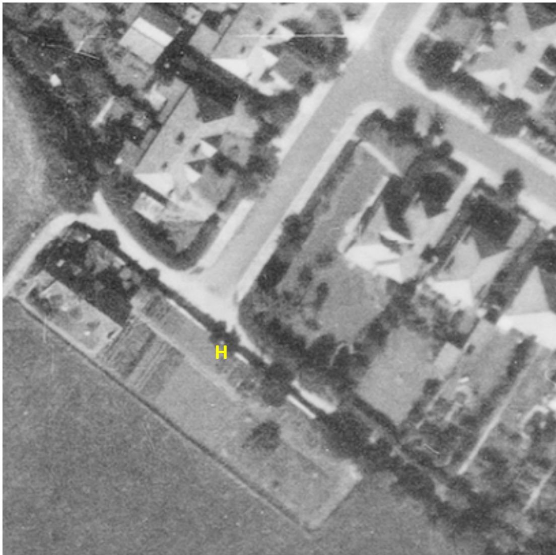
FIGURE 9: NO ACCESS AT POINT H, 1947
