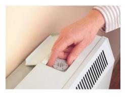
released can be increased by opening the internal damper valve and allowing air to enter the brick core.
