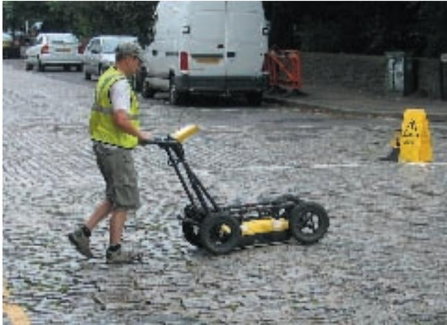
*Ground Penetrating Radar survey in progress*
