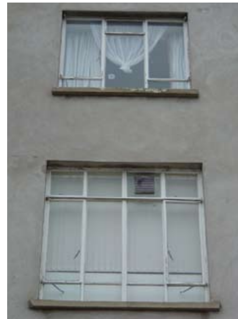
The use of inappropriate materials detracts from the original qualities of the elevations
