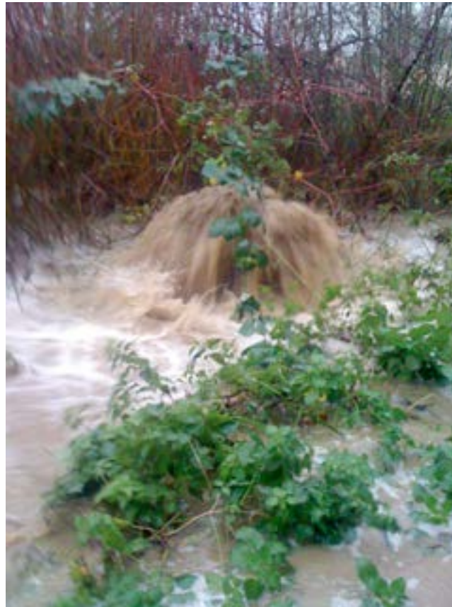
Surcharged surface water sewer in Withywood, November 2012
