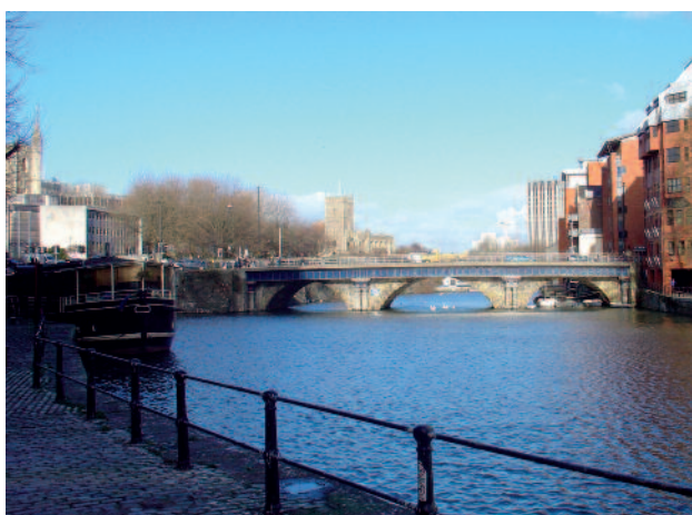
Figure 2: Looking towards Bristol Bridge from Welsh Back
